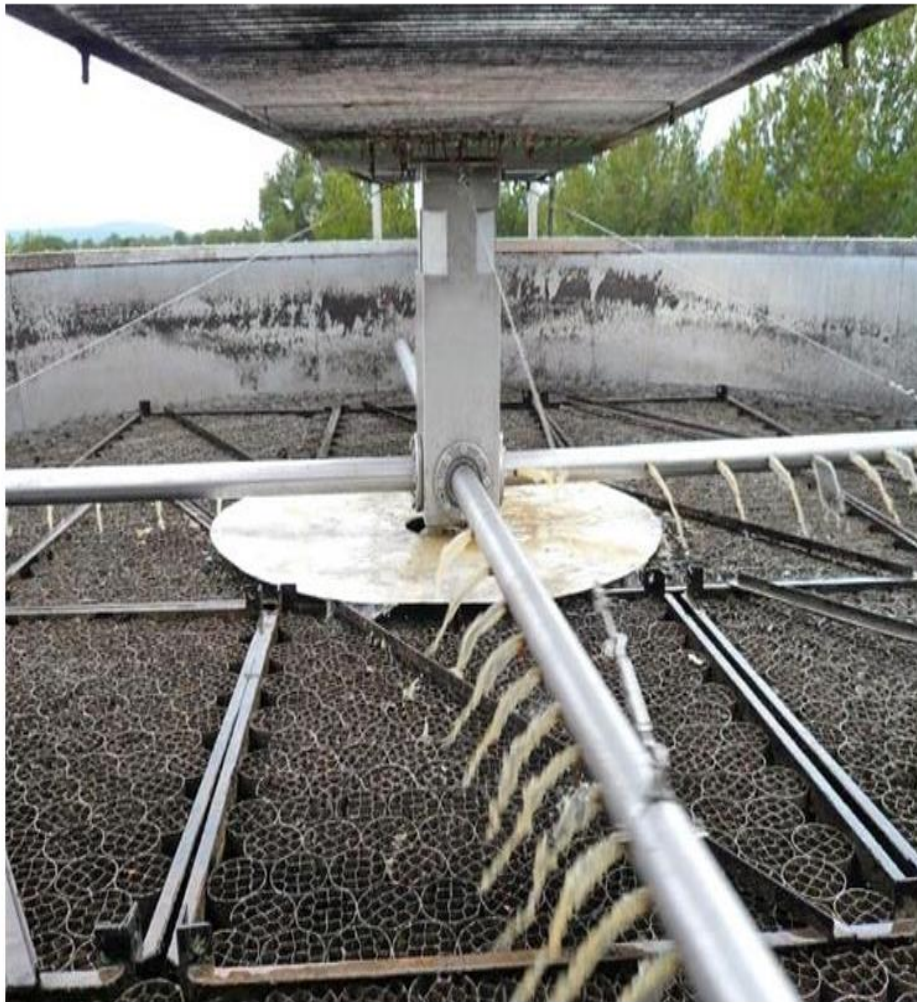
Figure 5: Operation of a bacterial bed
